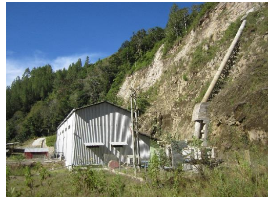
6MW Hydropower Plant in North Sumatra Province
