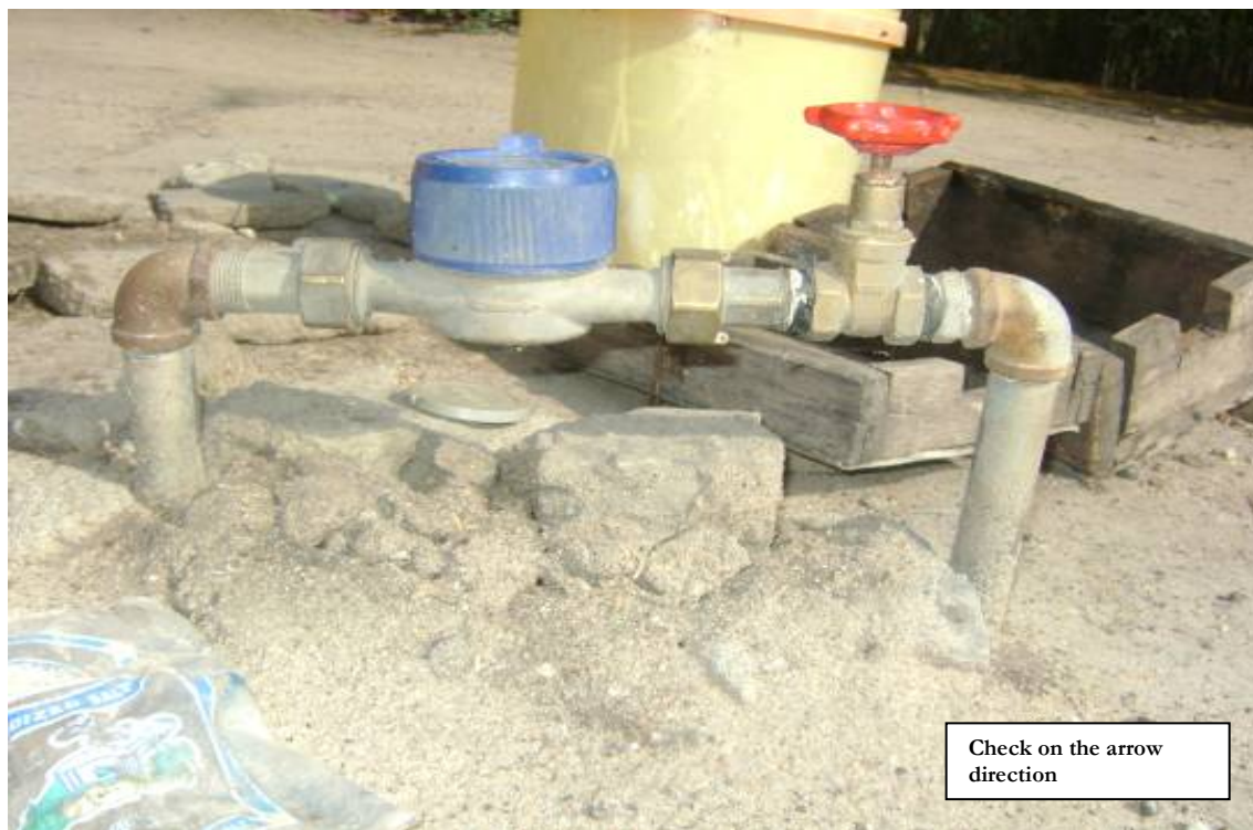
Figure 3: This is an example of a “reversed” meter. It has been tampered with so it can register a low reading.
