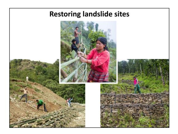
Landslide sites were rehabilitated using bioengineering, in combination with 'hard' measures like gabions where needed. This activity intensified after the 2015 earthquake caused many landslides. These sites were often at risk of further slides as a result of extremely heavy rainstorms.
