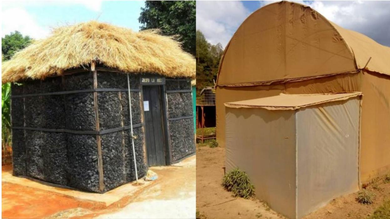
*Figure 2: Charcoal Cooler (Left); Screenhouse (Right)*
