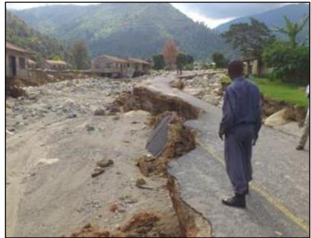
IMAGE 4. PAVED ROAD WASHED OUT BY FLOOD IN KASESE
