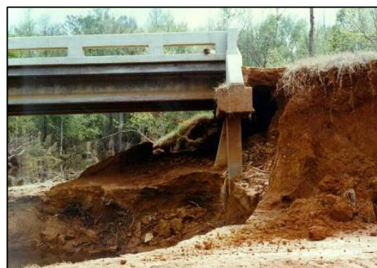
IMAGE 5. ILLUSTRATION OF BRIDGE SCOUR UNDERMINING BRIDGE SUPPORTS.
